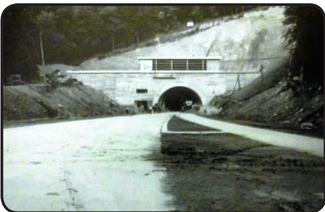
In the Summer of 1940, the roadbed has been cemented and the tunnel entrance completed with the exhaust fan second story built.
