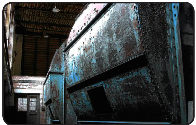
Inside the second story fan room with huge fans still there in 2007 used to rid the vehicle exhausts when in use.
