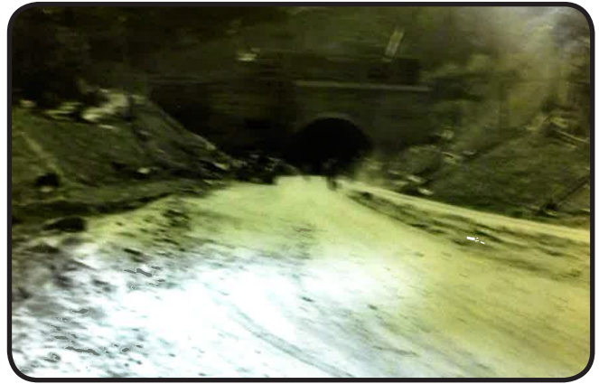
The entrance to Sideling Hill has been built and the road bed for the turnpike leveled.
